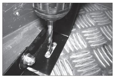
NOTE - Beware of electric cables when drilling holes
